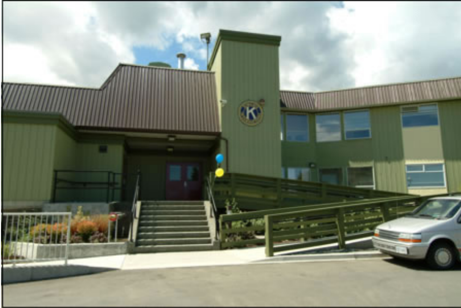
Exterior of building
